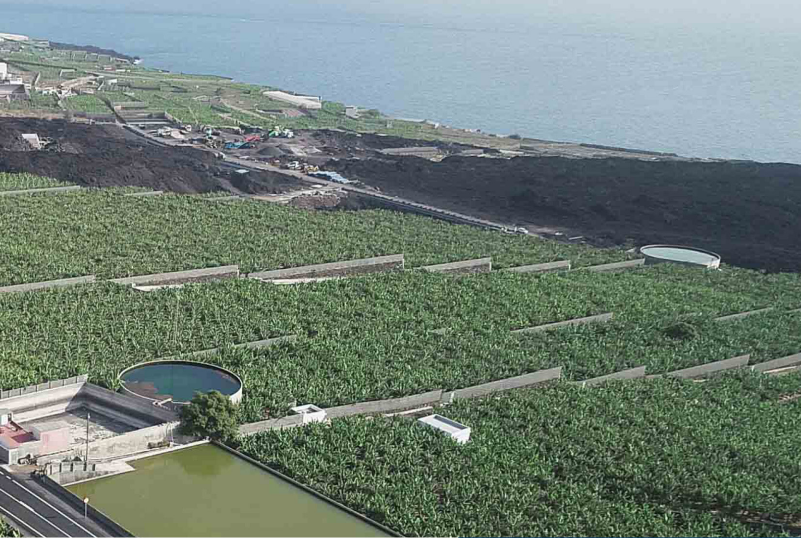
LA PALMA ROAD, BUILT ON THE LAVA, SPAIN - © DRAGADOS
