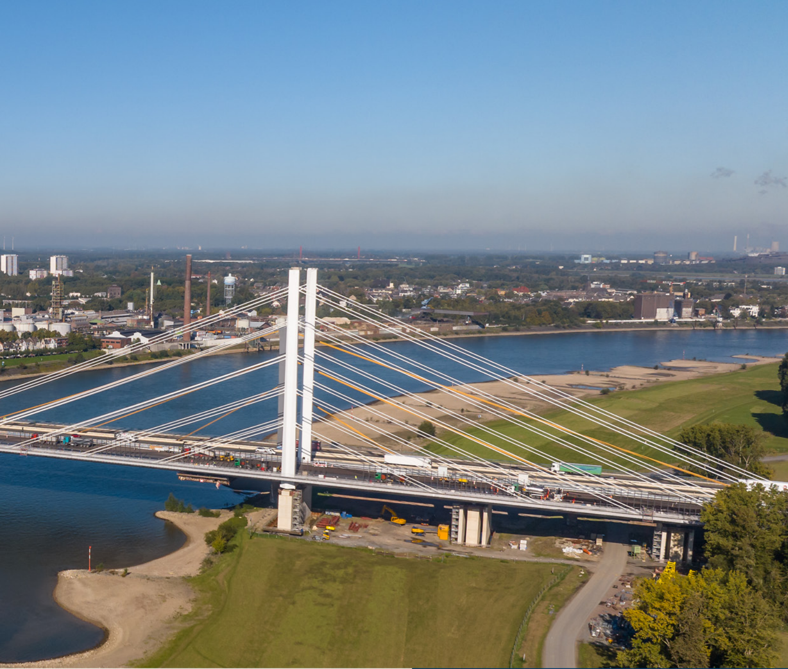
A40 BRIDGE OVER THE RHINE IN DUISBURG, GERMANY - © HOCHTIEF
