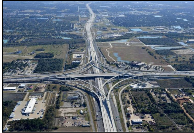
New managed toll lanes constructed in the median of SH 288
