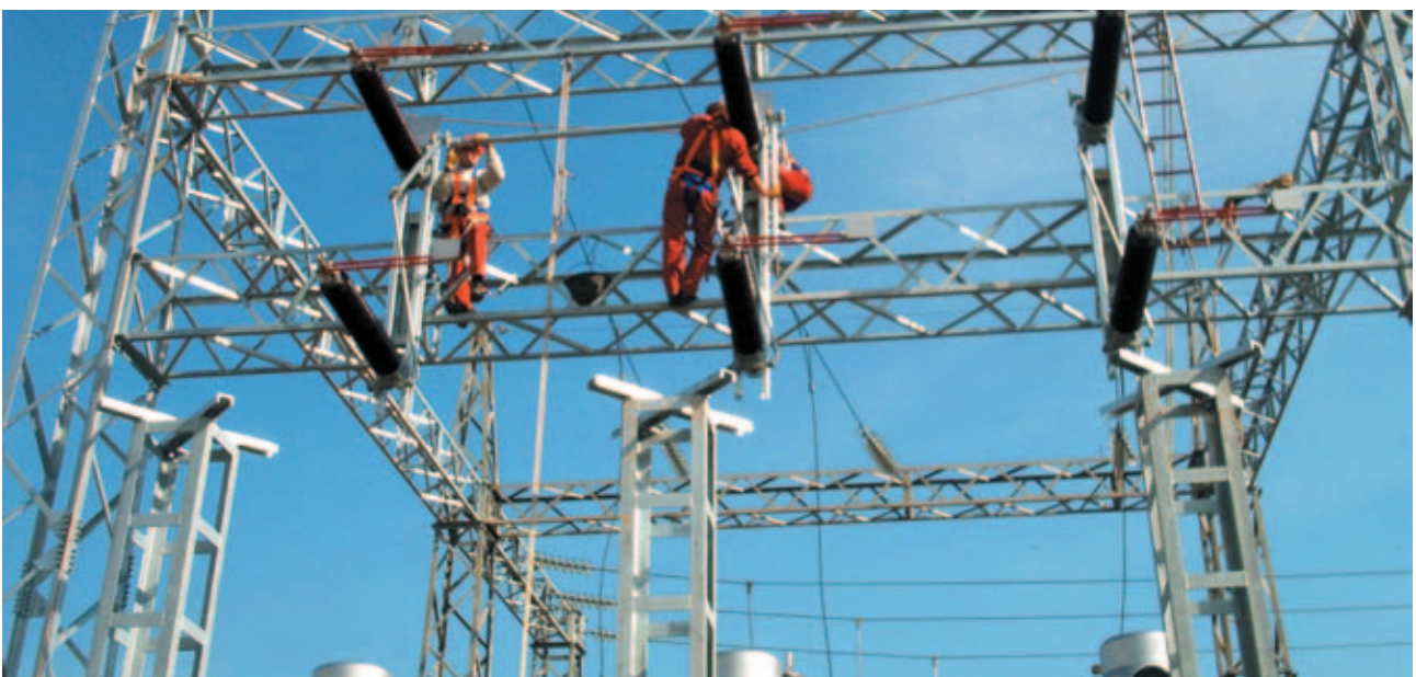
Maintenance of the electrical grid
