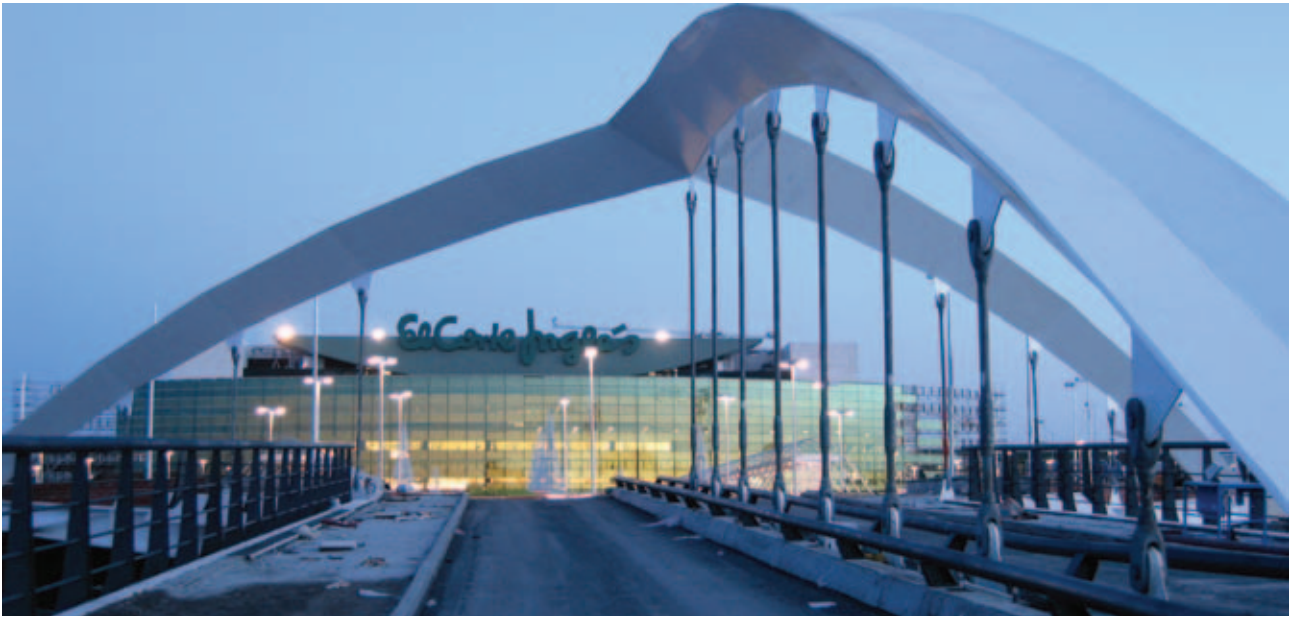
Three-support bridge in Sanchinarro (Madrid)
