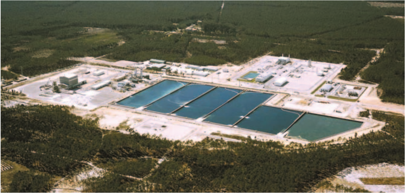
Underground storage of natural gas, Carricho (Portugal)
