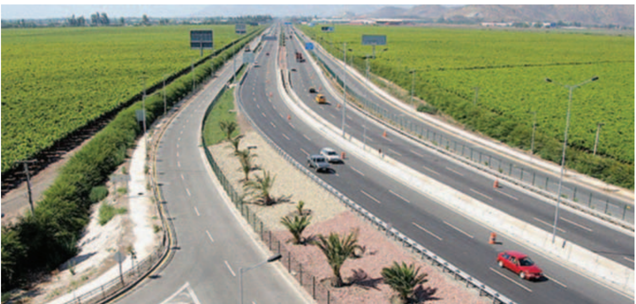
Santiago-Valparaiso motorway (Chile)
