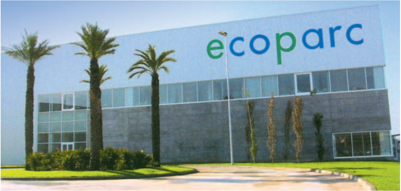
Solid urban waste treatment plant in Barcelona
