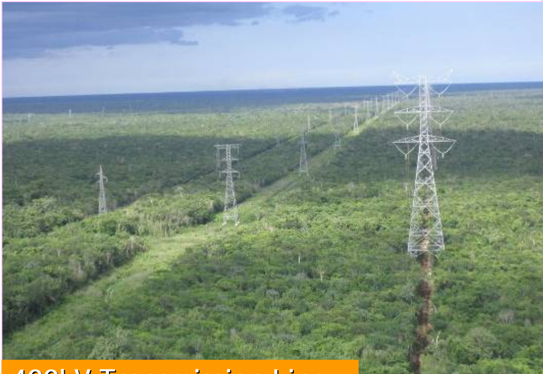
400kV Transmission Line Maya Riviera (Mexico)
