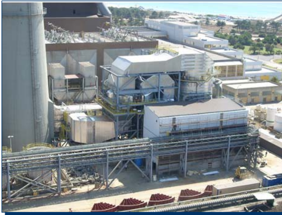
Thermal power station in Sines (Portugal) 95% Sulphur deletion and 50% Dust elimination 1.200.000 Nm 3 /h gas treatment
