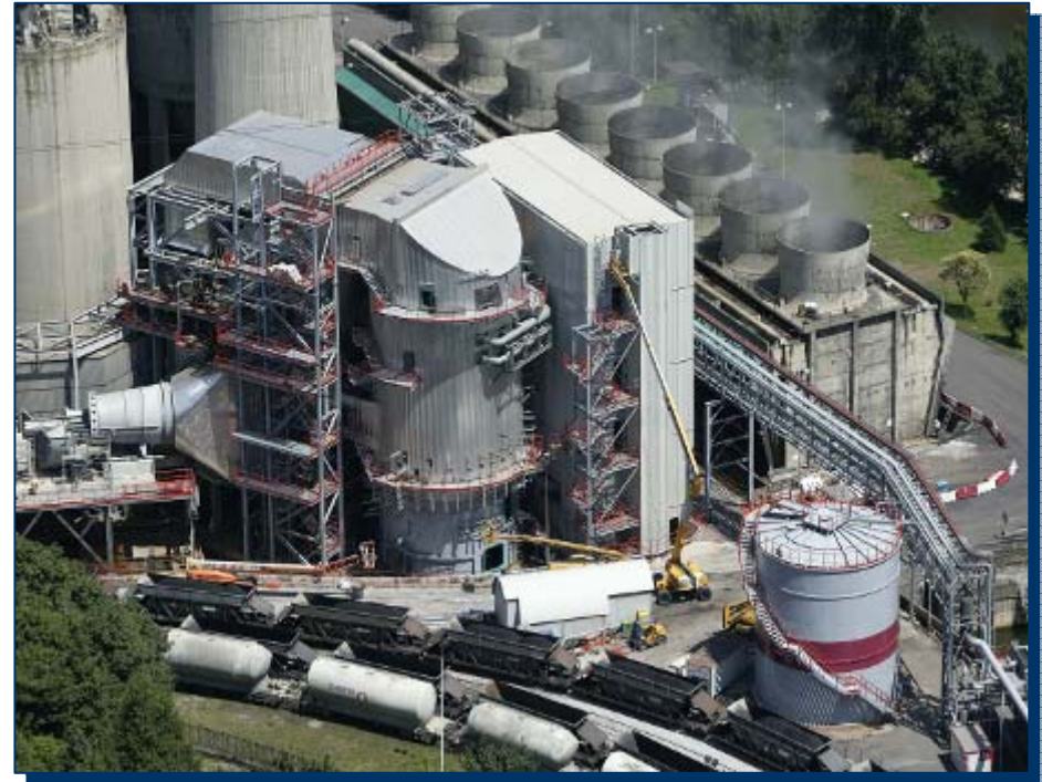
Soto III Thermal power station (Asturias) 95% Sulphur deletion 50% Dust deletion 1.330.000 Nm 3 /h gas treatment
