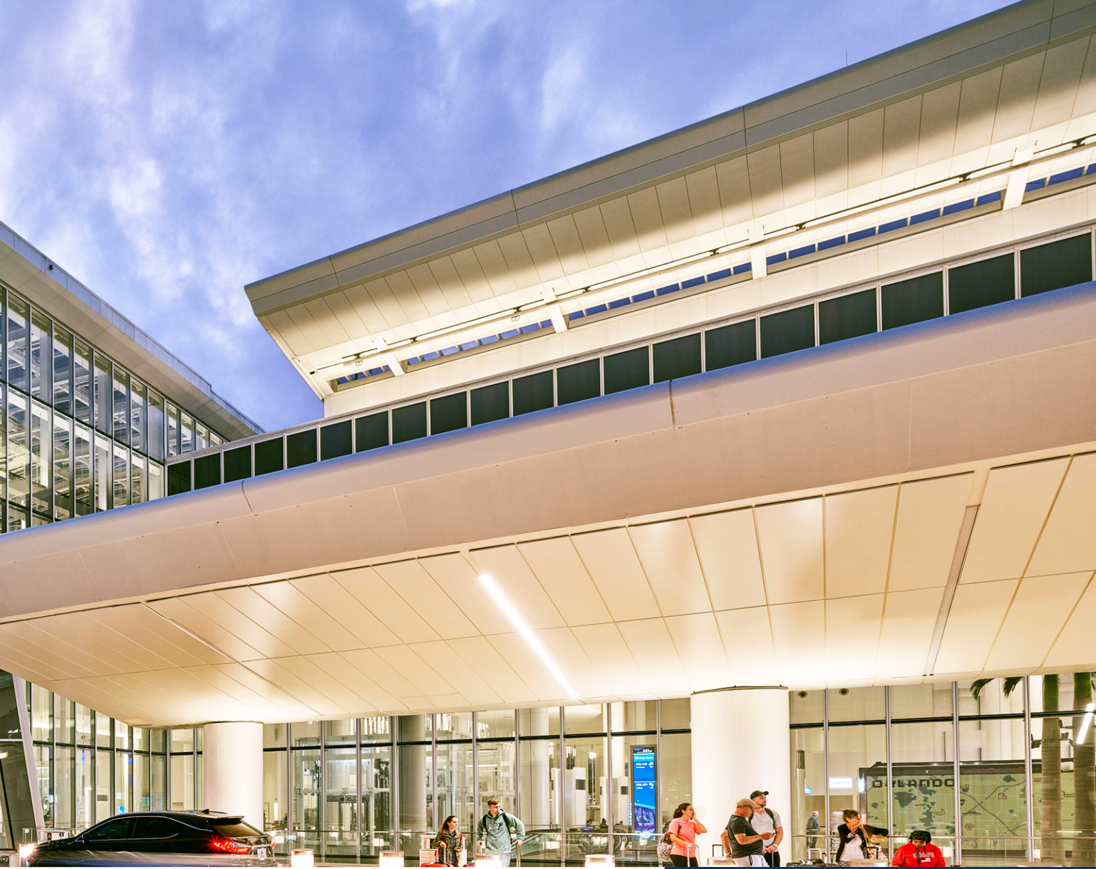
ORLANDO INTERNATIONAL AIRPORT, USA - © TURNER
