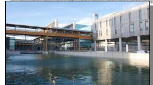
Treatment plant in Marseille
