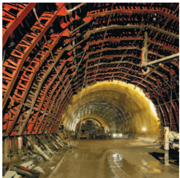
Tunnel in Niévares (Asturias)
