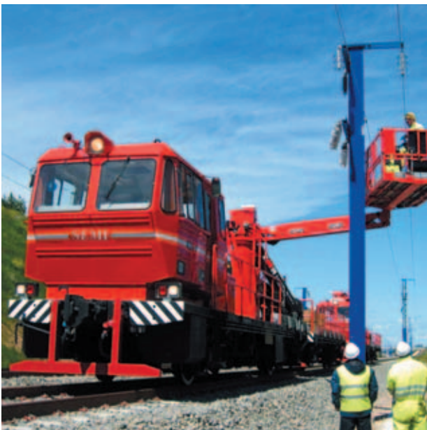
Maintenance of railway electrical grid
