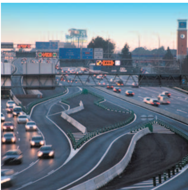
VAO bus control systems on the N-VI (Madrid)
