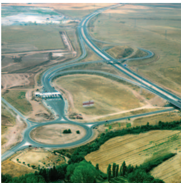
Radial 2 motorway in Madrid
