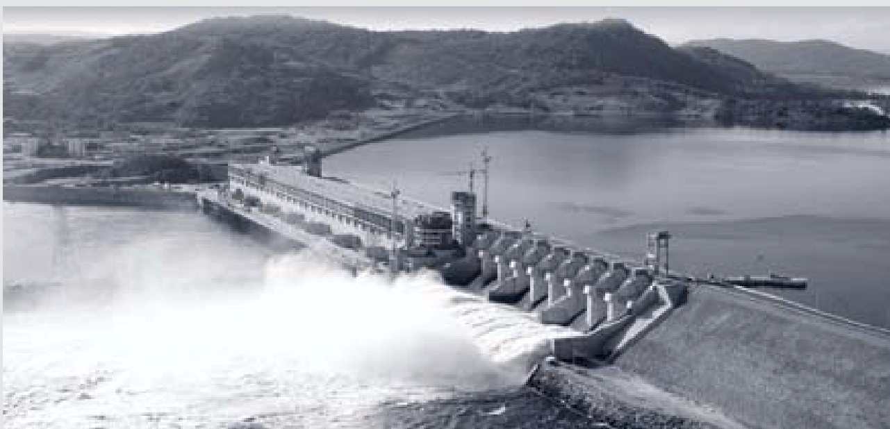
Dam in Caruachi (Venezuela)
