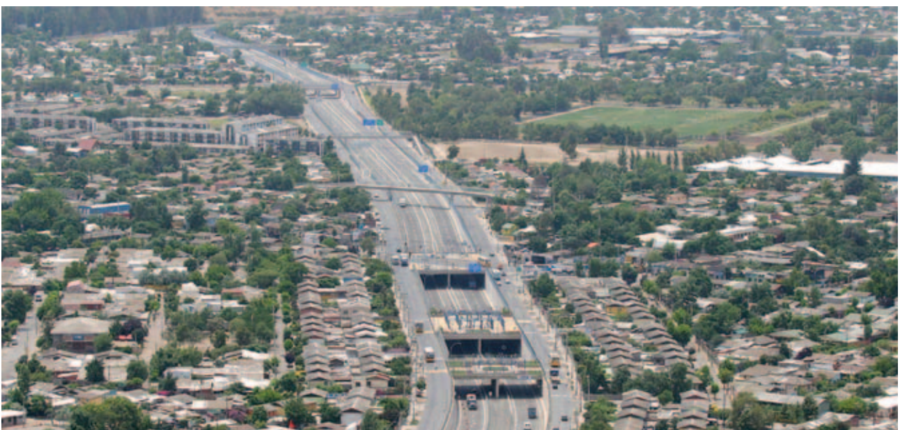
Central motorway (North-South urban system) in Chile
