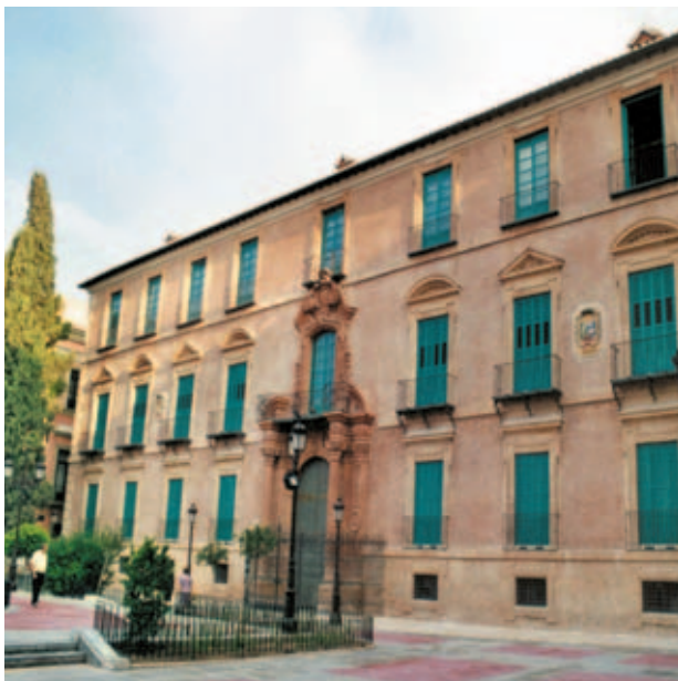
Rehabilitation of the Episcopal Palace of Murcia
