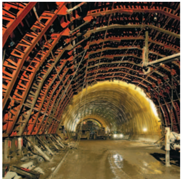
Tunnel in Niévares (Asturias)
